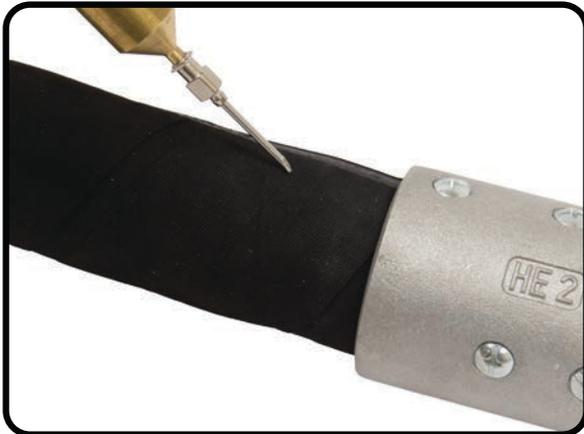
**STEP 1:** Insert the needle into the blast hose at a 45° angle about 1" before the nozzle holder. Always insert the needle with the sharp edge down and the open side toward the nozzle. Push the needle far enough into the blast hose for the tip to pierce the inner wall.
